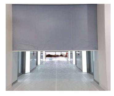
Fire containment systems prevent the spreading of smoke from one zone to another. NAFFCO curtain comprises of flexible heat resistant fabric with fire integrity up to 240mins.\* The tube contains a DC electric motor which holds the curtain retracted at ceiling level at all times and deploys upon the receipt of fire alarm signal. The bottom bar ensures safe and controlled descent of the curtain with gravity fail safe.
